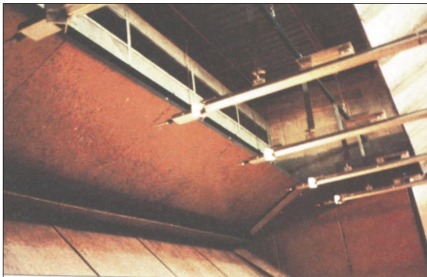
Exhaust grilles at the apex of the bullet trap.
