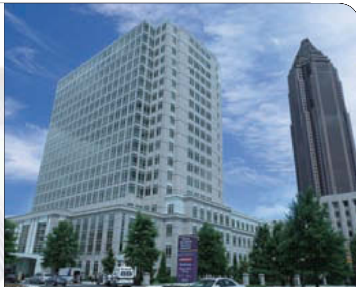
Emory University Midtown Hospital in Atlanta saved money by changing filters based on performance instead of a calendar date.
