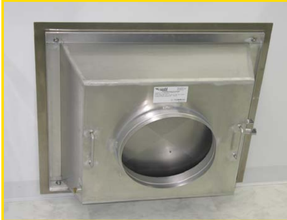
Top photo: Pharmaseal Exhaust Housing installed in a cleanroom wall offers an aesthetically pleasing room side appearance. Bottom photo: Same unit with testing shroud mounted on the Pharmaseal frame for overall filter efficiency testing from within the room.
