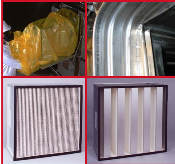
Top left: Workers are protected during filter service by containment process of changing filters within a bag.
